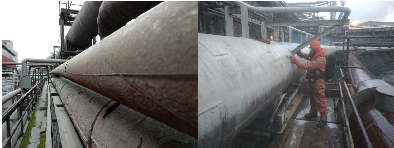
Figure 2. Mounting of optical fiber for pipeline monitoring
